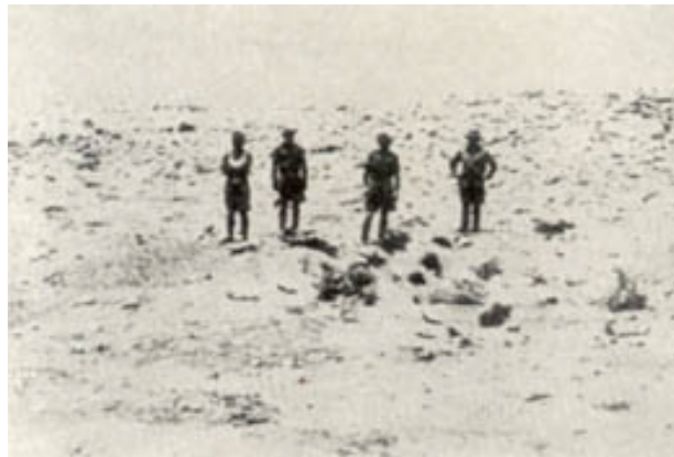
FIGURE 57. In front of the men is a vehicle, dug in and camouflaged to blend with the background. Spoil is slightly mounded around the excavation and gradually sloped to meet existing terrain level. Both vehicle and spoil are covered with a light screen made of chicken wire and cloth, over which is spread sand, a few rocks, and some brush.
